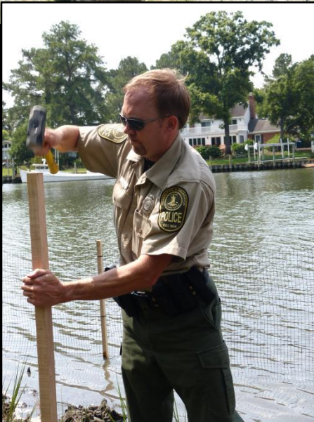
State Park staff helped with the project
